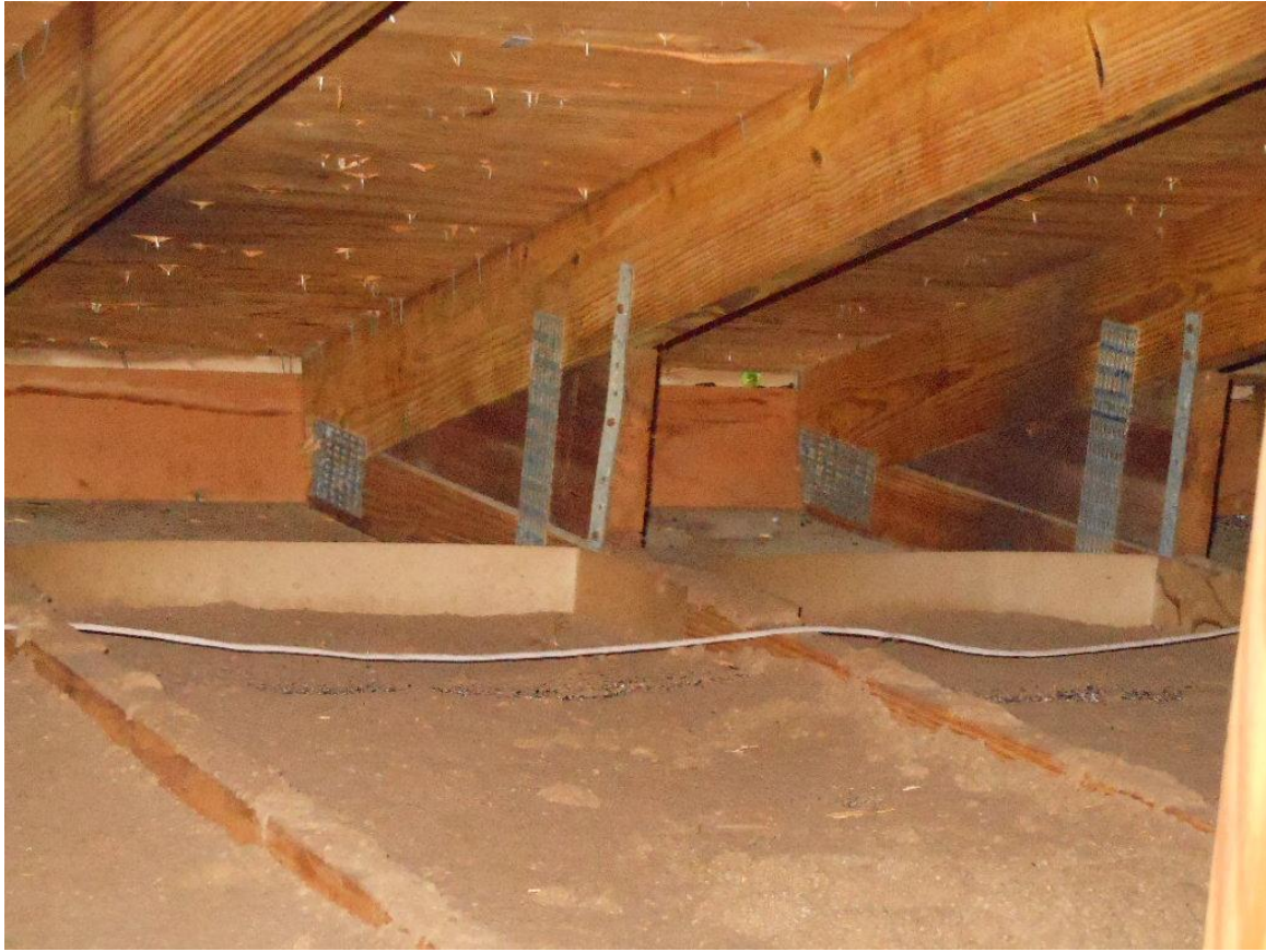
Roof to wall clips
