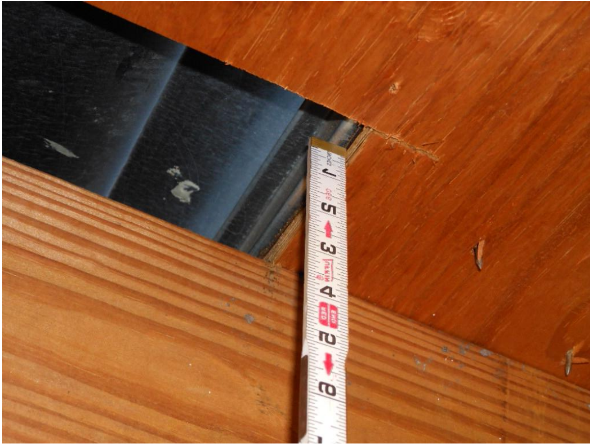
Roof deck staples
