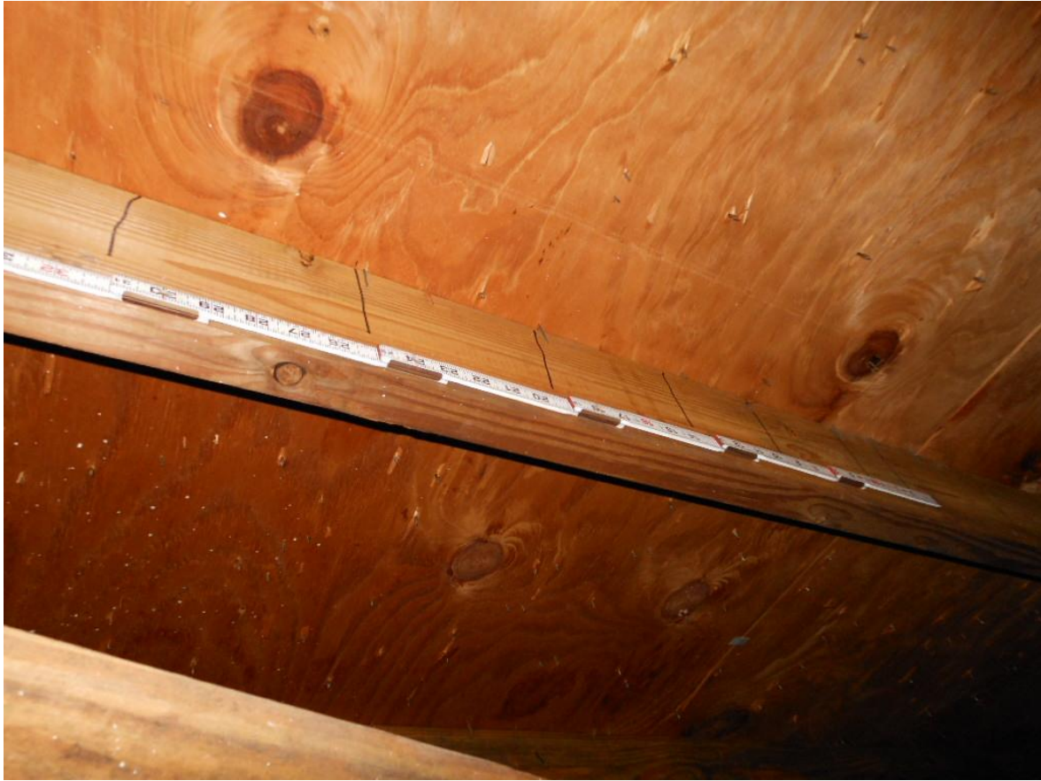
Roof deck staples
