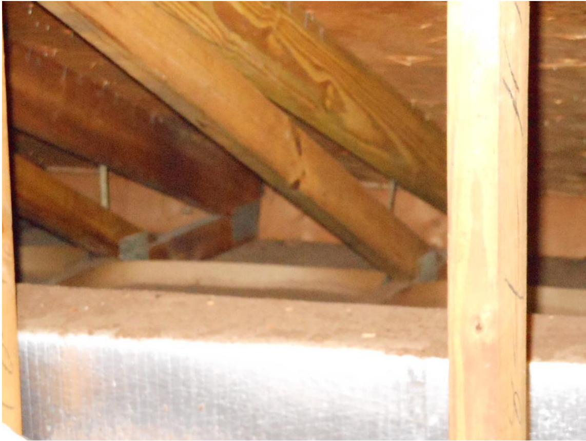
Roof to wall clips
