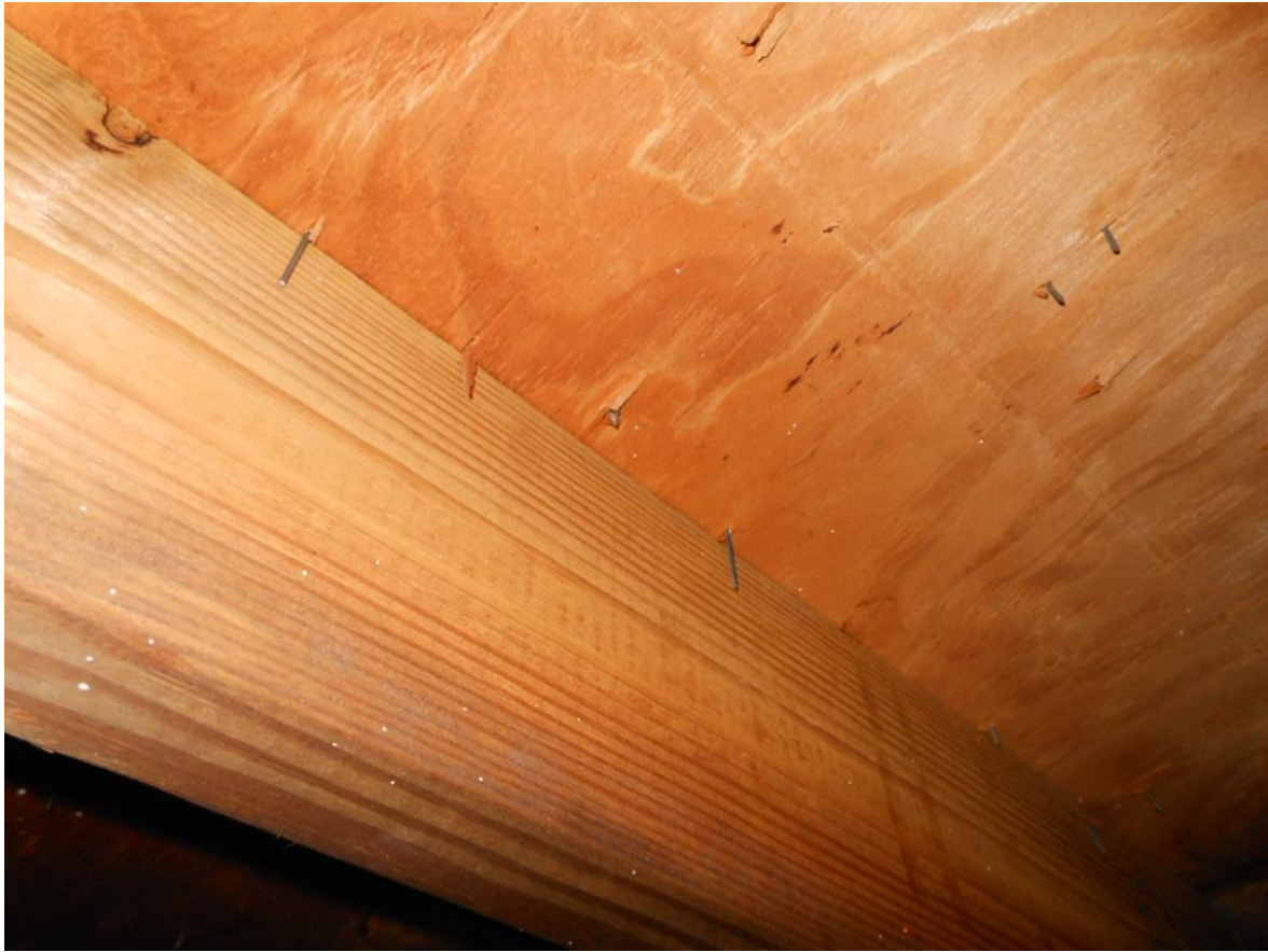
Roof deck staples
