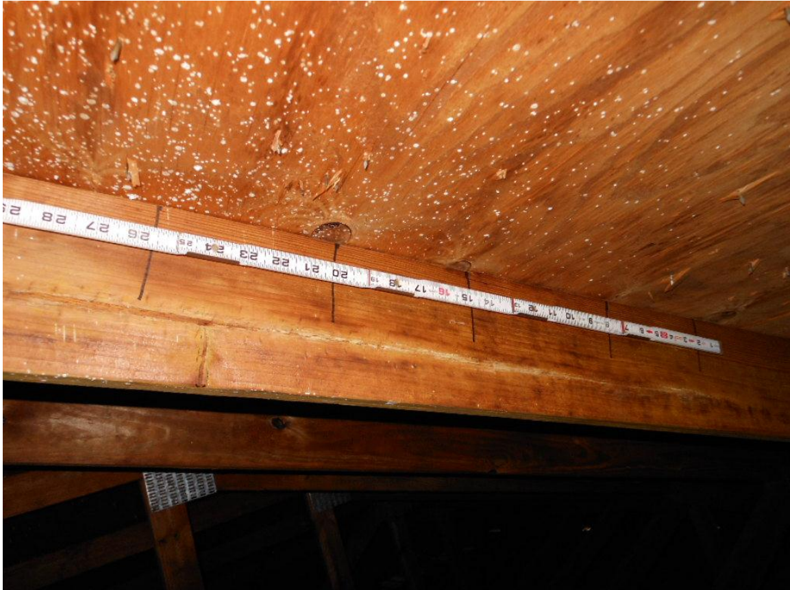
Roof deck staples
