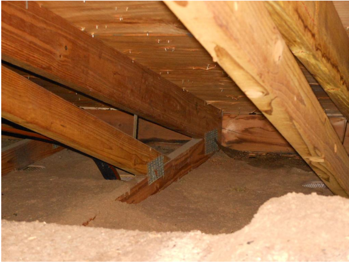
Roof to wall clips
