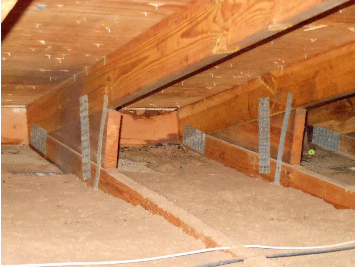
Roof to wall clips
