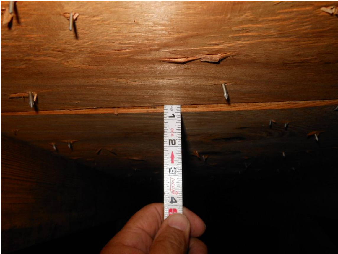
Roof deck staples
