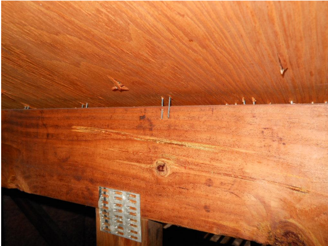
Roof deck staples
