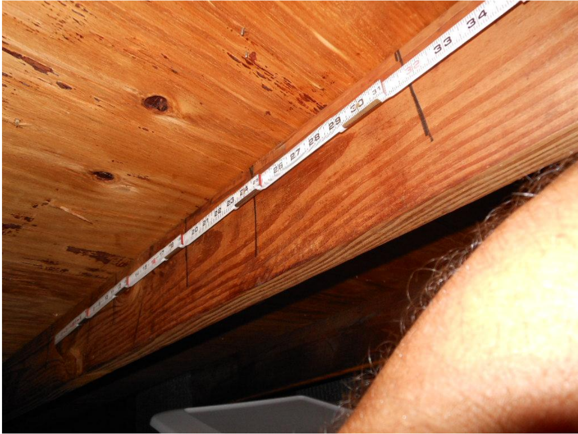
Roof deck staples
