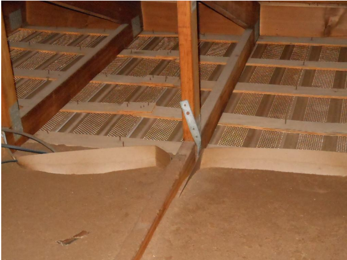
Roof to wall clips
