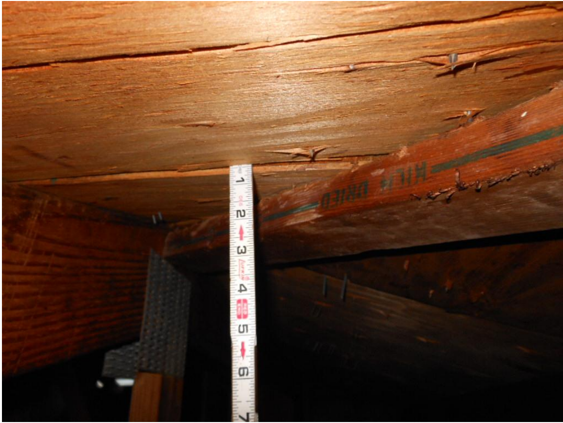
Roof deck staples
