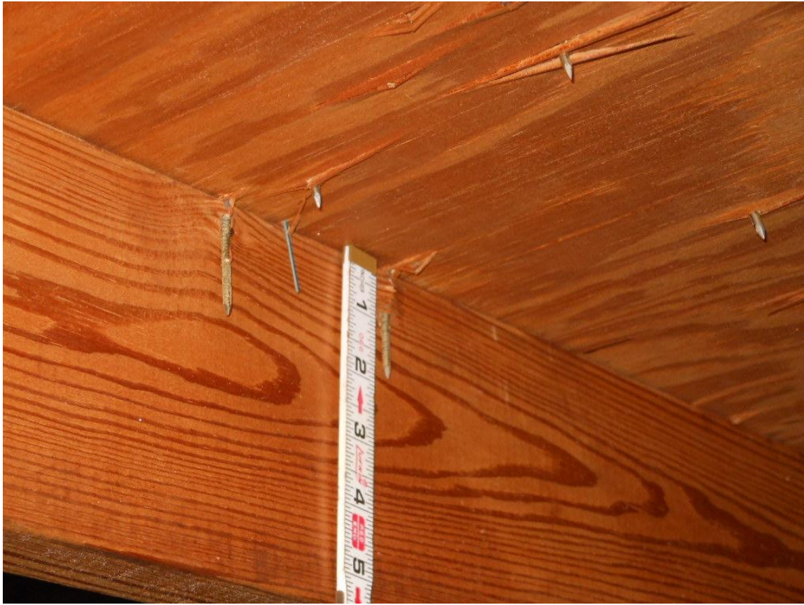
Roof deck 8d nails 6x6
