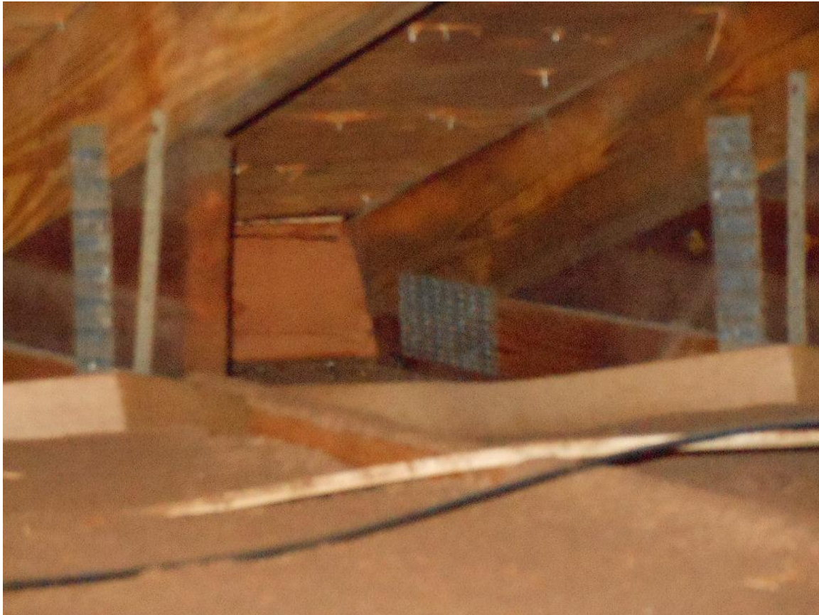
Roof to wall clips
