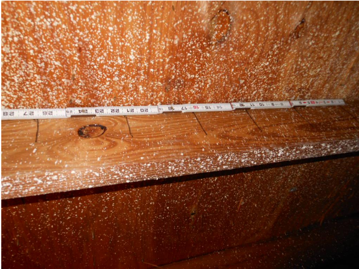
Roof deck 8d nails 6x6
