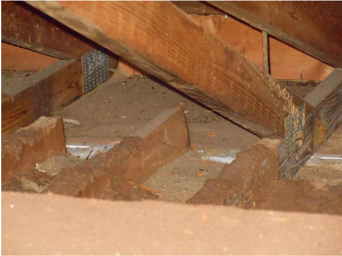
Roof to wall clips
