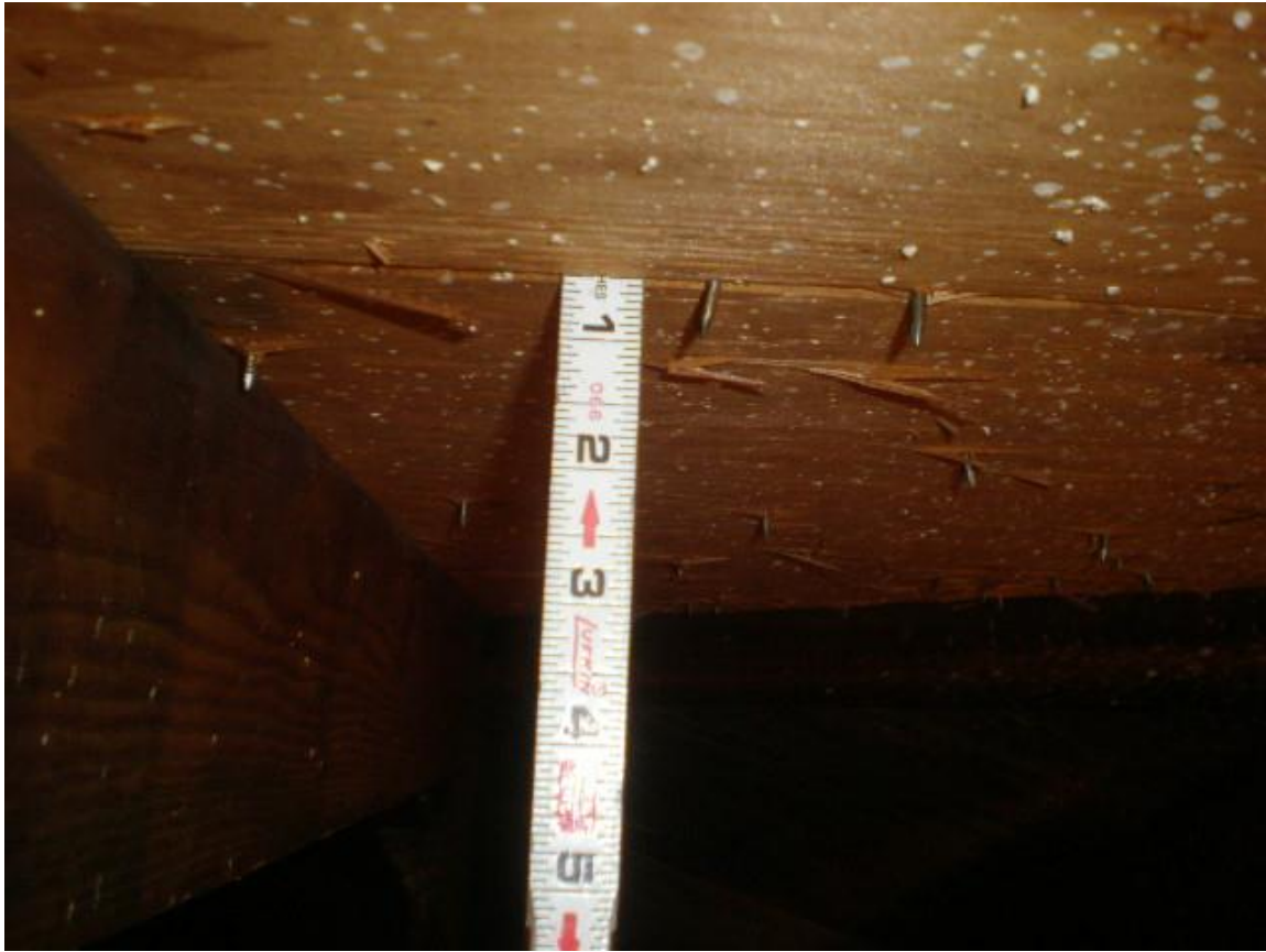
Roof deck staples
