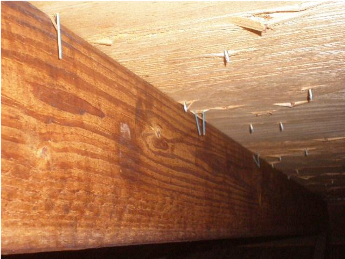
Roof deck staples
