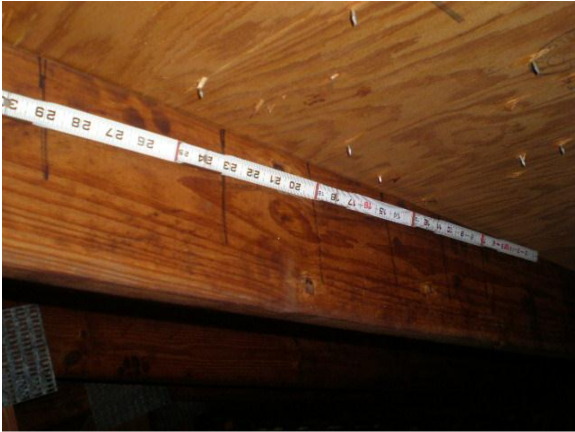
Roof deck staples
