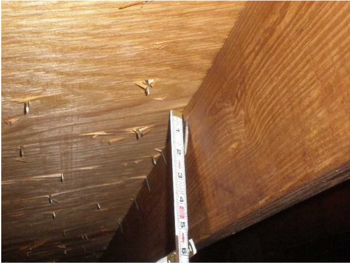
Roof deck 8d nails 6x6
