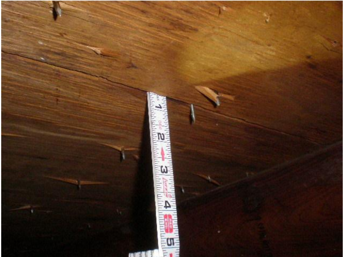
Roof deck 8d nails 6x6
