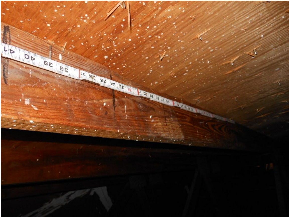
Roof deck 8d nails 6x6
