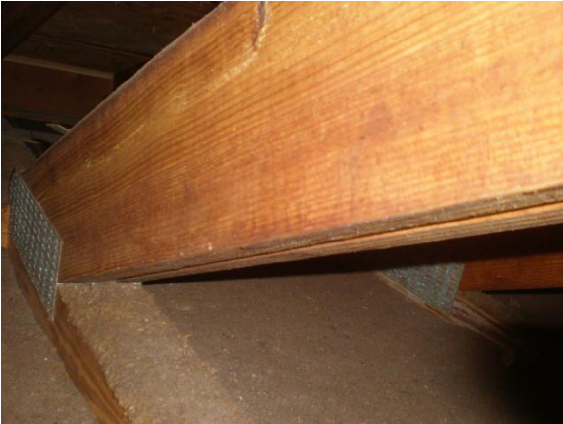
Roof to wall clips
