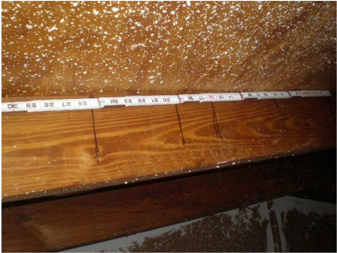
Roof deck staples
