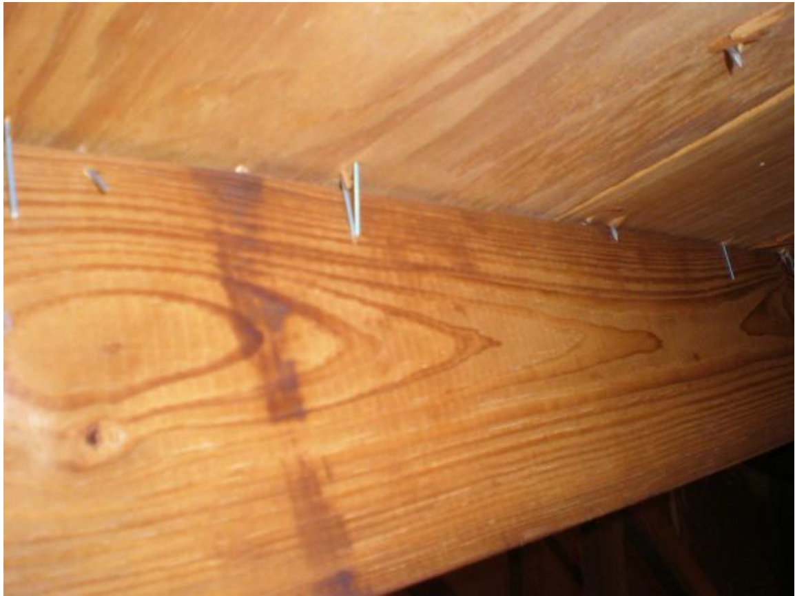
Roof Deck staples
