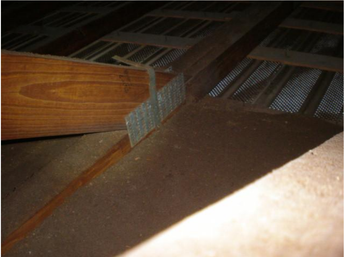
Roof to wall clips
