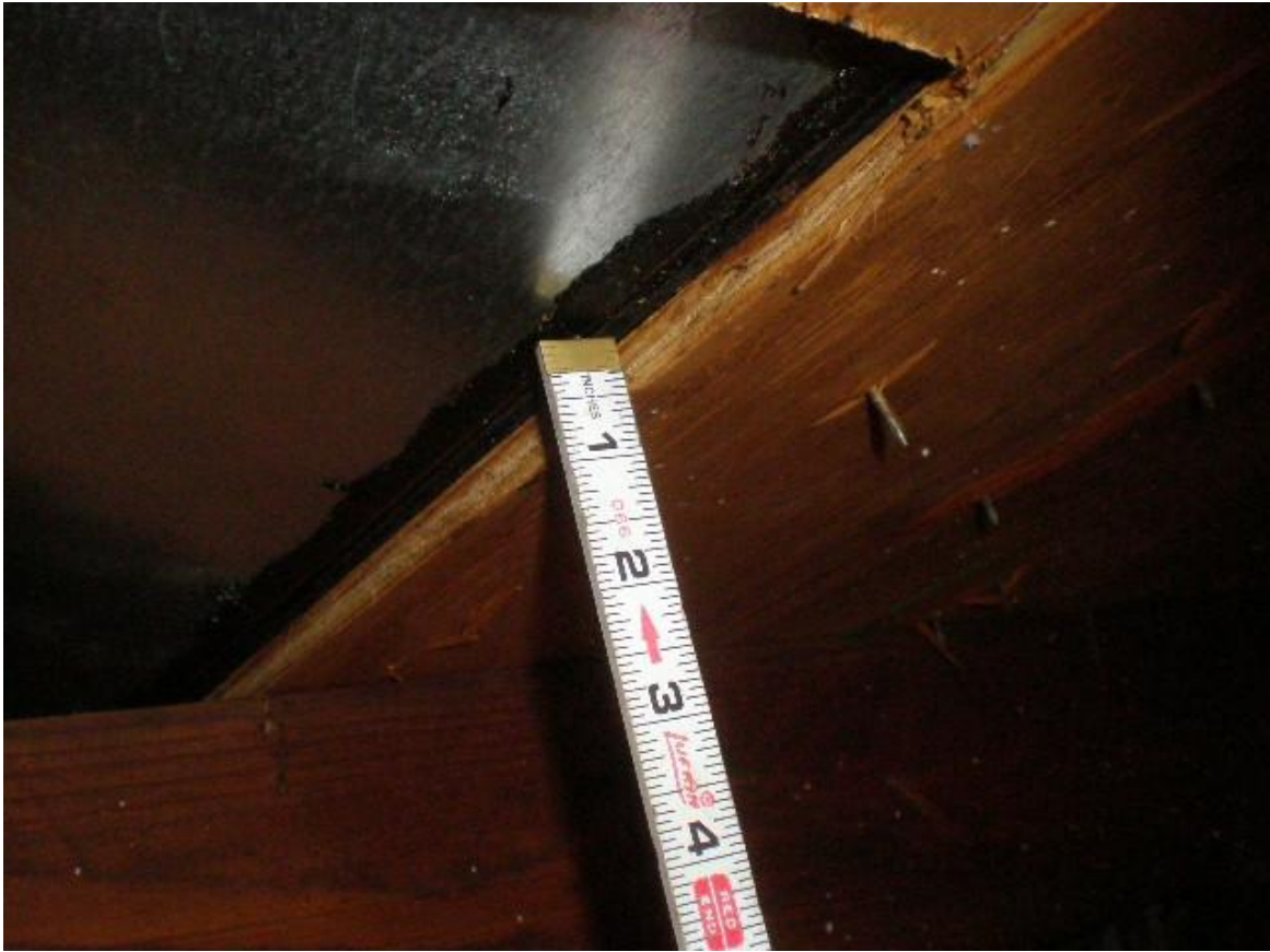
Roof deck staples
