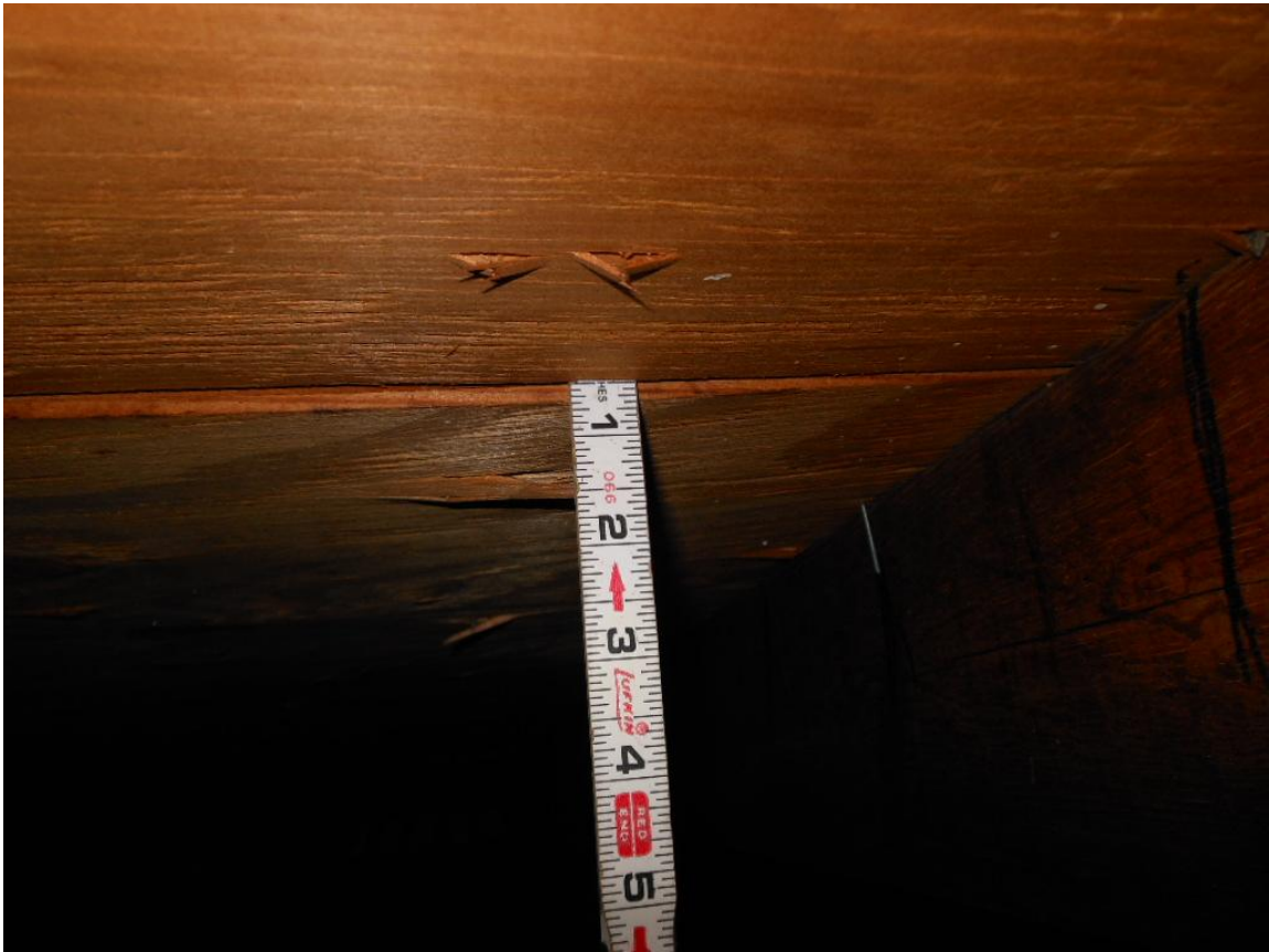
Roof deck staples
