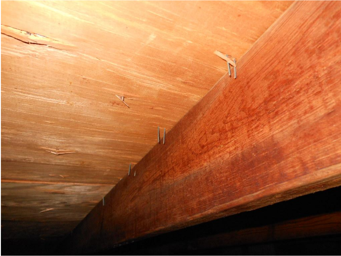
Roof deck staples
