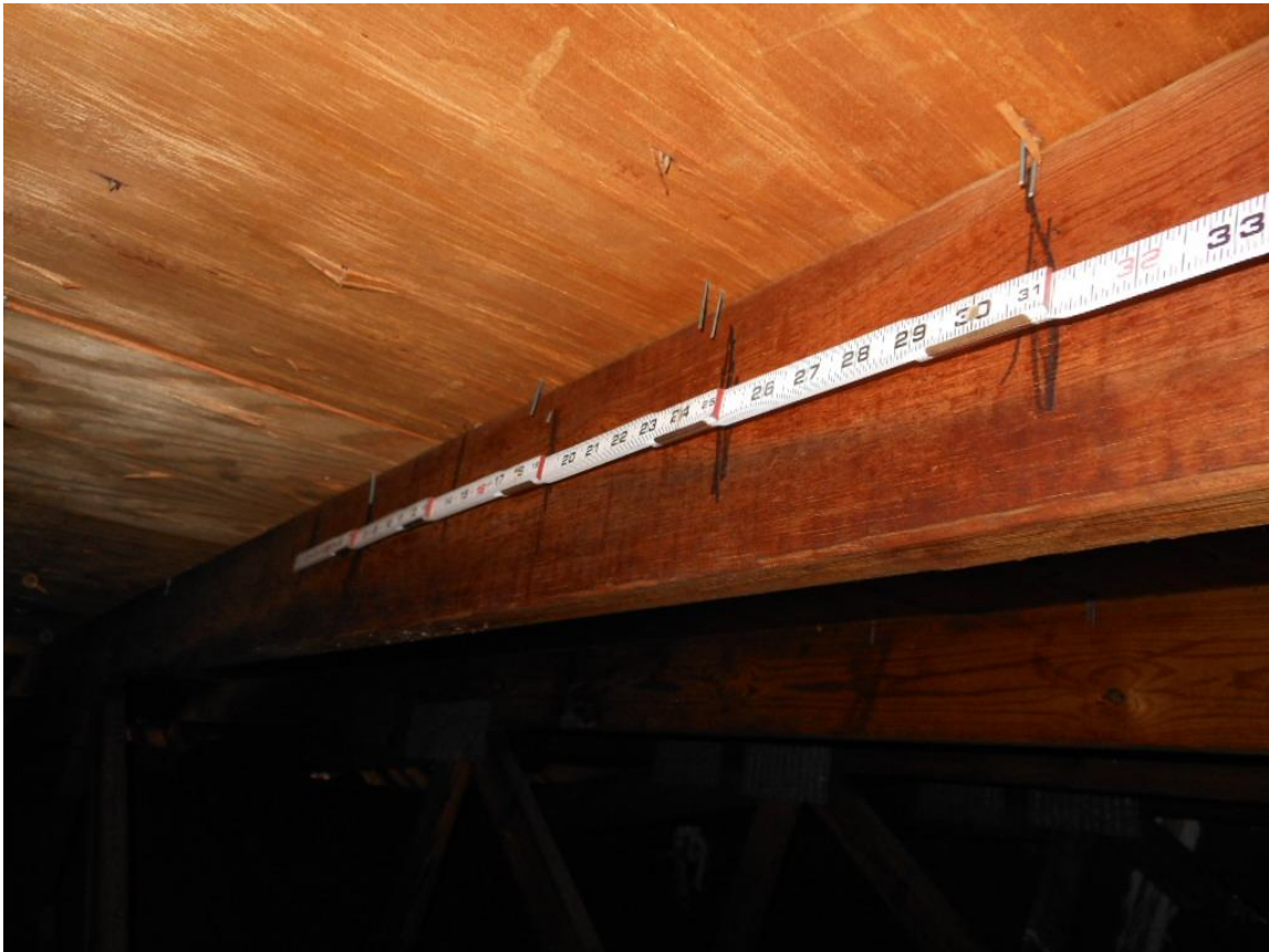
Roof deck staples
