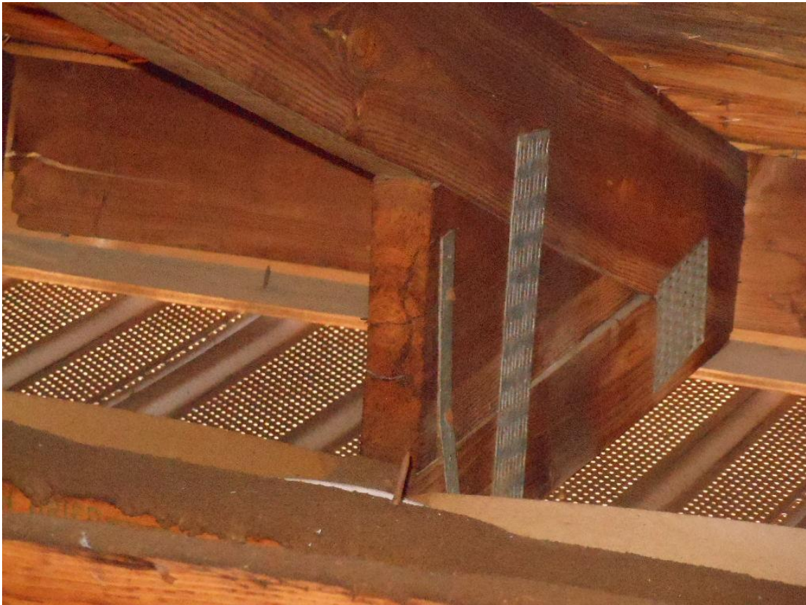
Roof to wall clips
