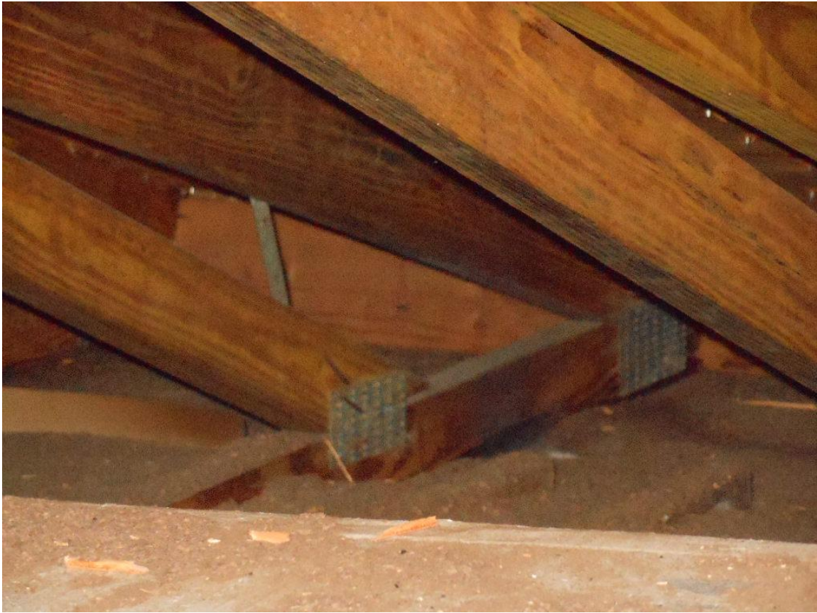
Roof to wall clips
