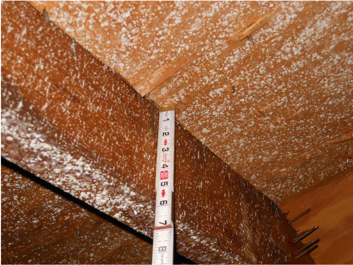
Roof deck 8d nails 6x6
