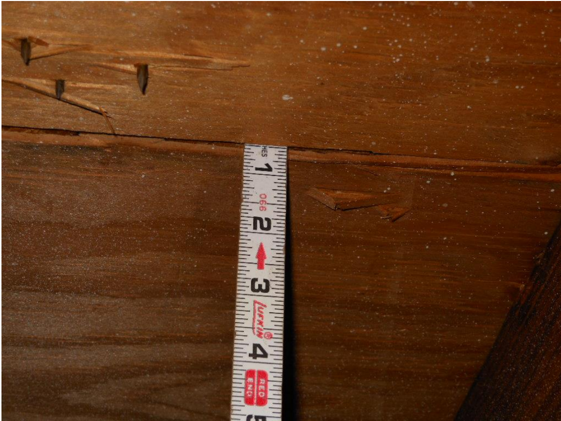
Roof deck 8d nails 6x6
