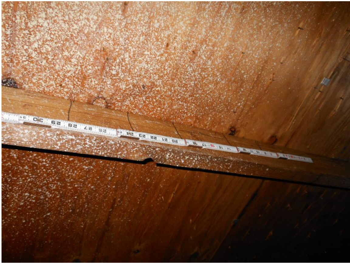
Roof deck 8d nails 6x6
