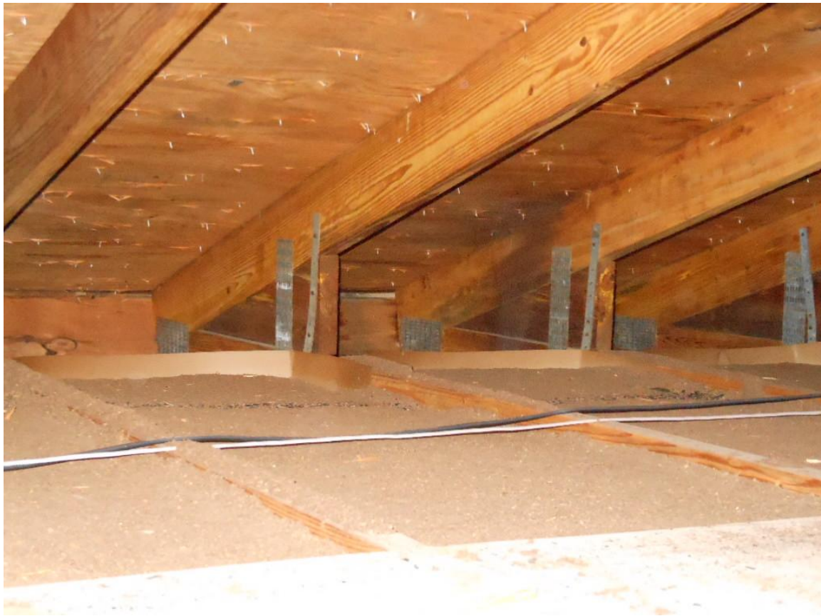
Roof to wall clips
