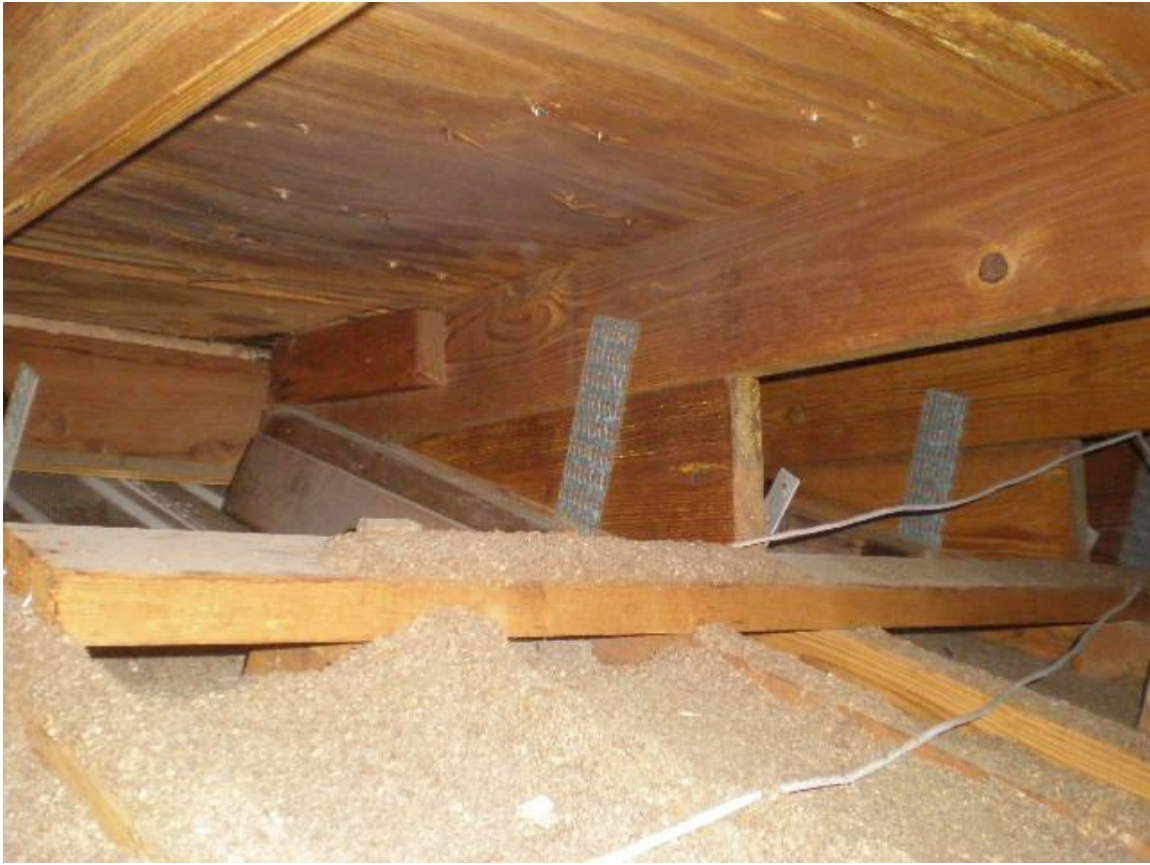
Roof to wall clips
