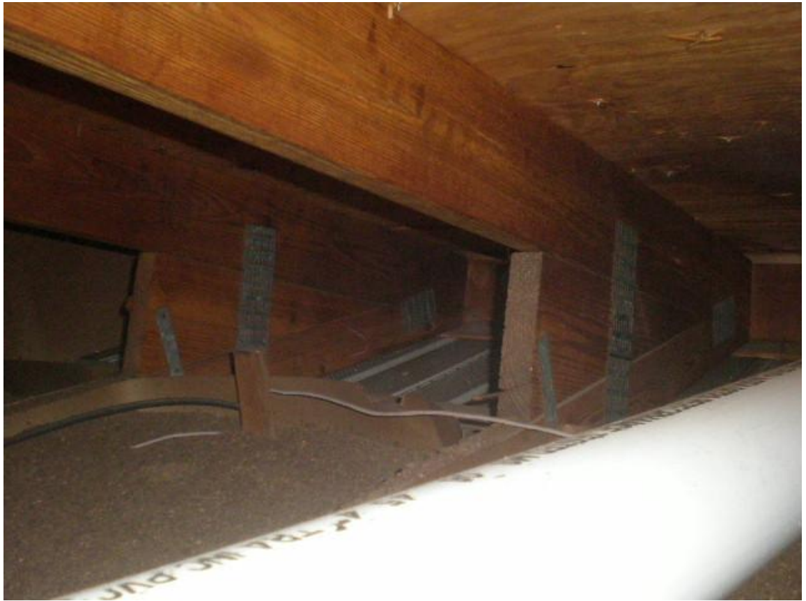
Roof to wall clips
