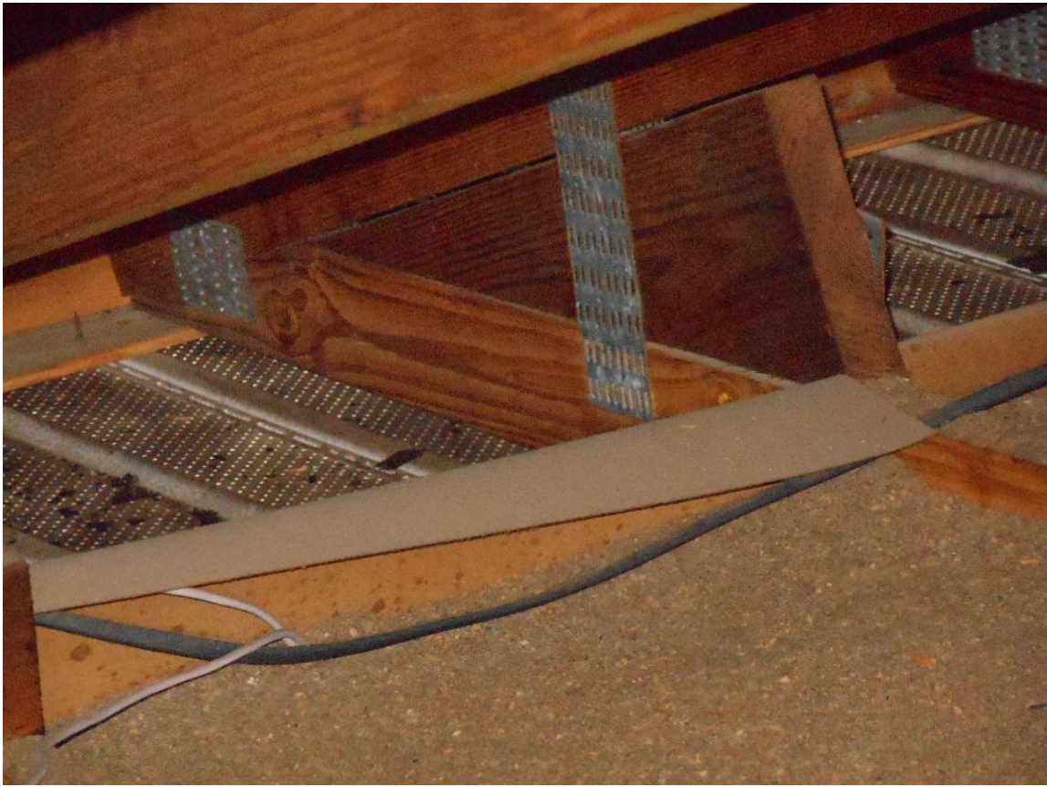
Roof to wall clips
