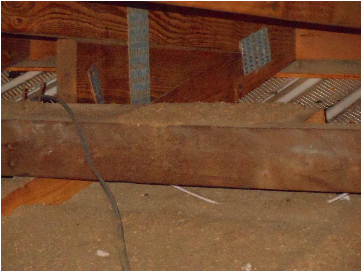
Roof to wall clips
