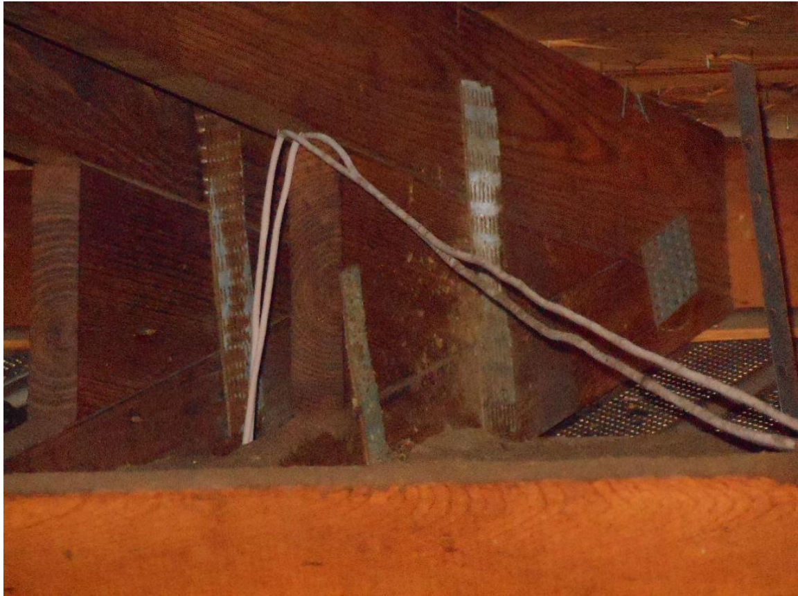
Roof to wall clips
