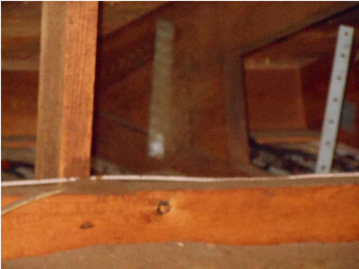
Roof to wall clips
