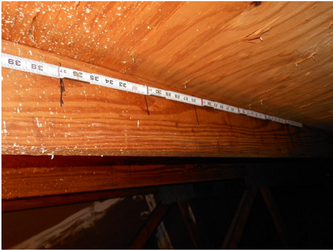
Roof deck 8d nails 6x6
