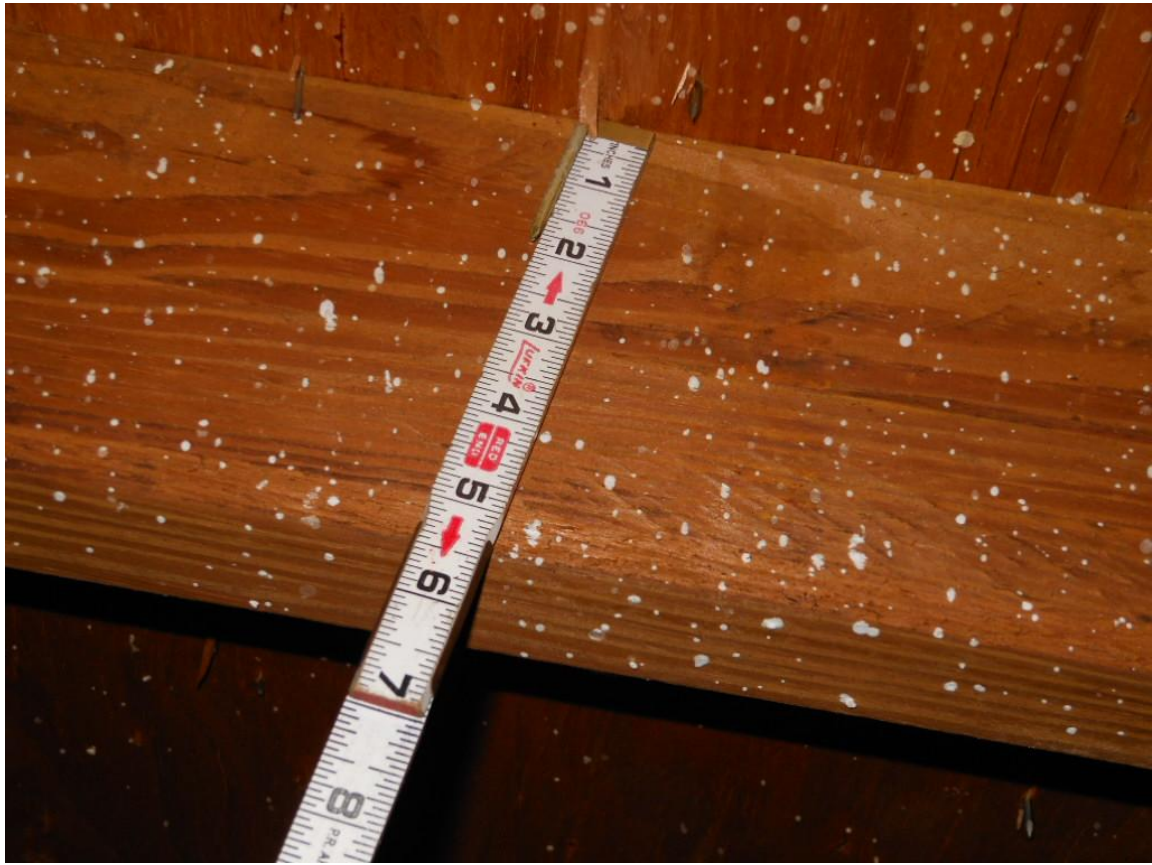
Roof deck 8d nails 6x6
