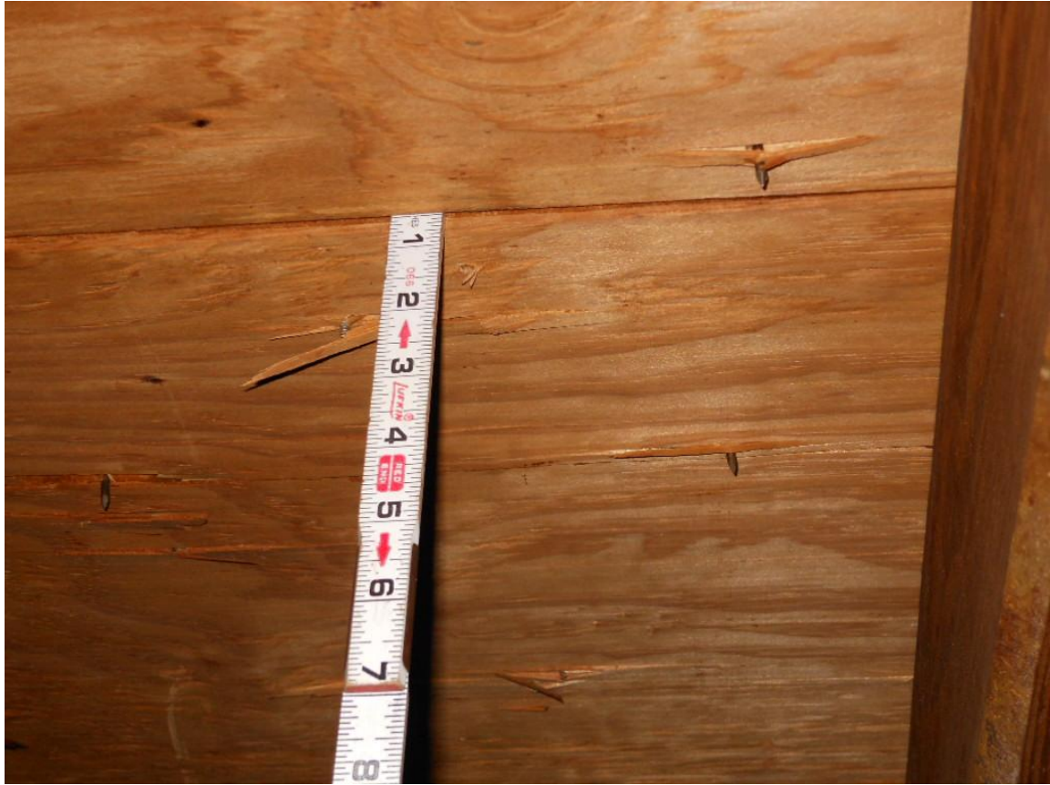
Roof deck 8d nails 6x6
