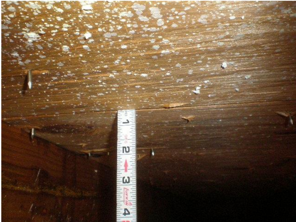
Roof deck staples
