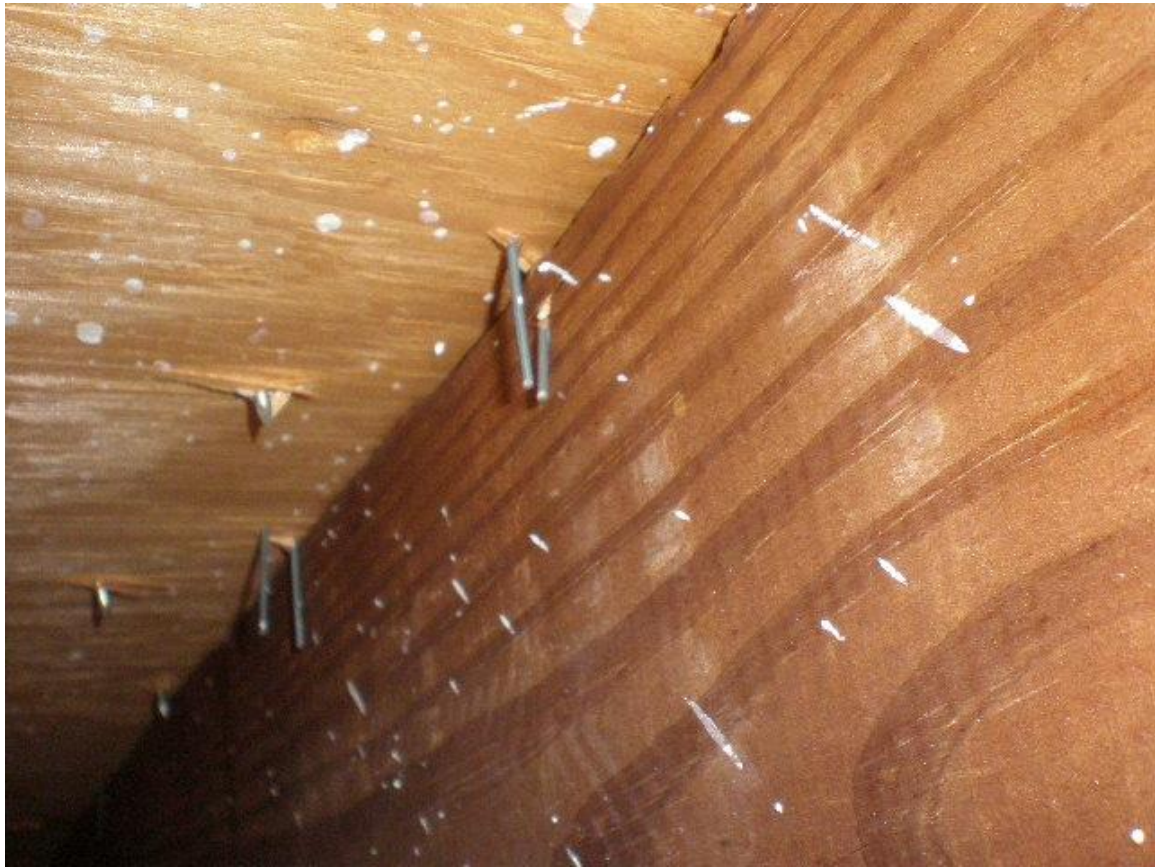
Roof deck staples
