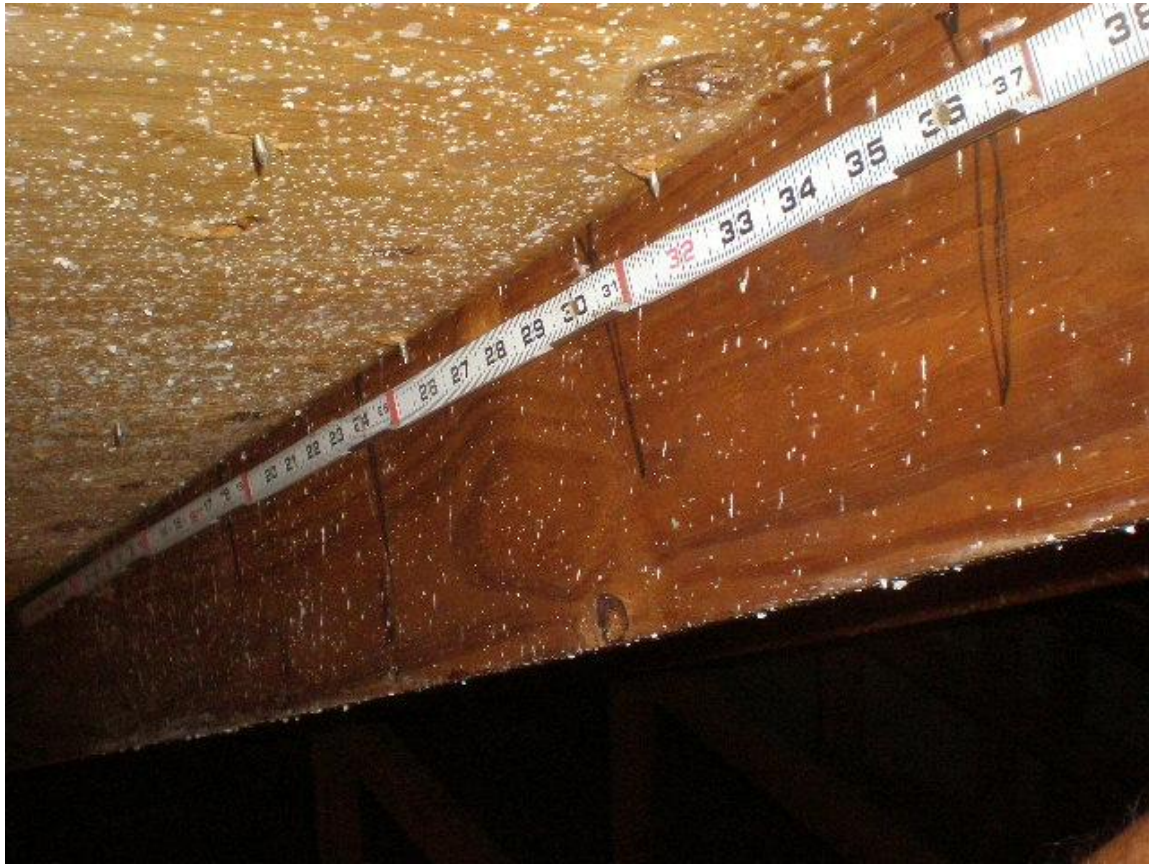
Roof deck staples
