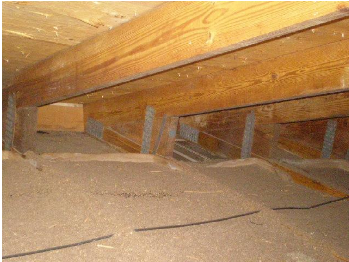
Roof to wall clips
