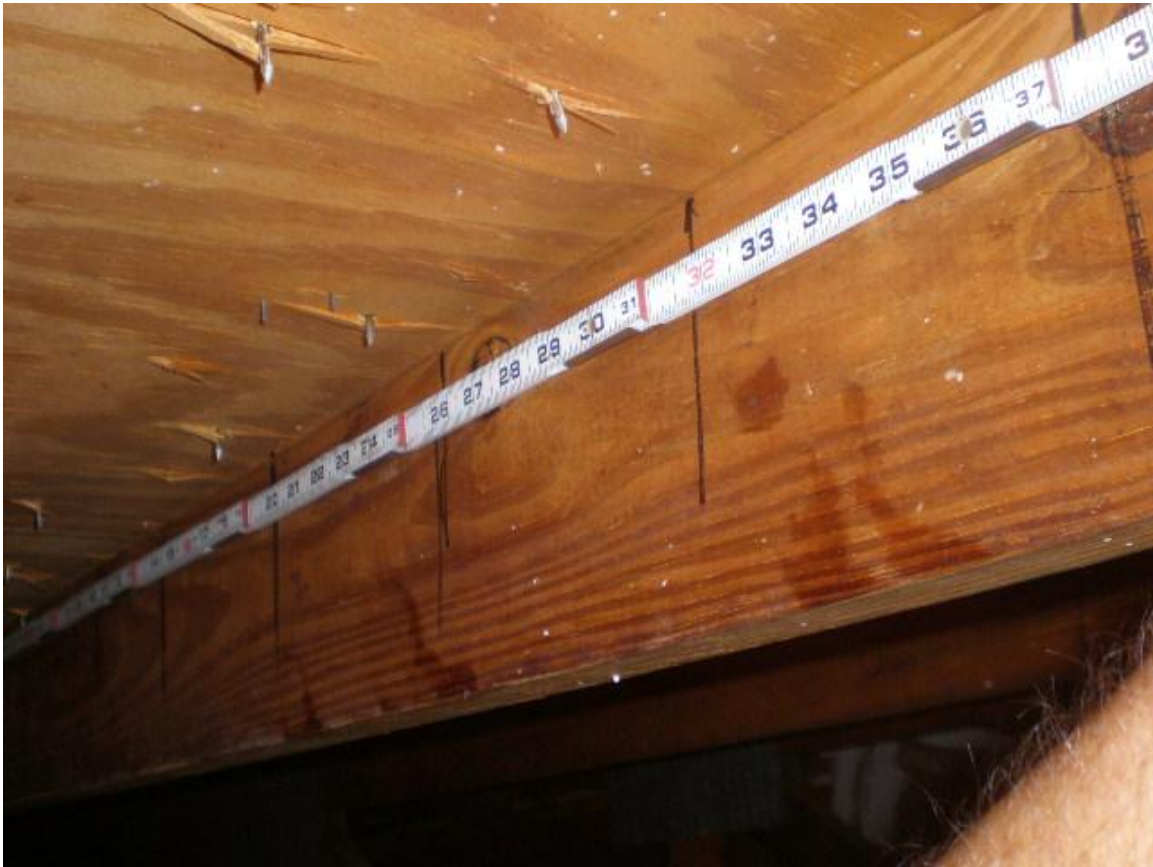
Roof deck 8d nails 6x6
