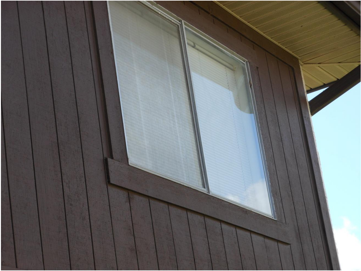
Unprotected openings
