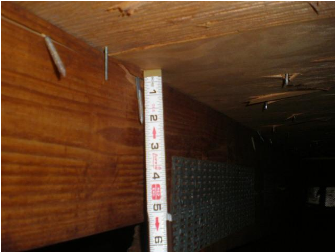
Roof deck 8d nails 6x6
