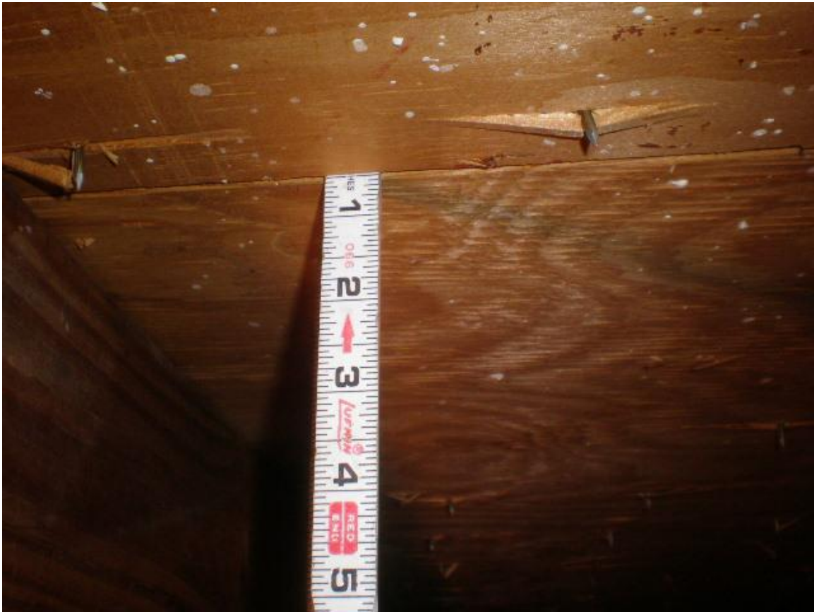
Roof deck 8d nails 6x6
