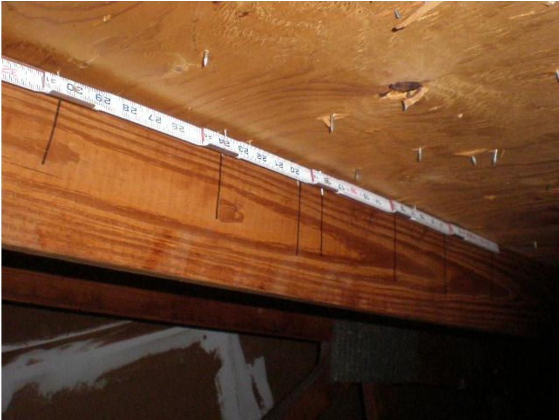
Roof deck staples
