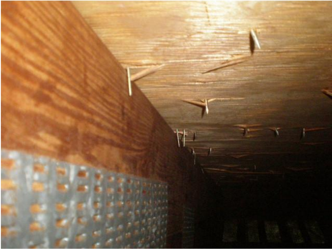
Roof deck staples
