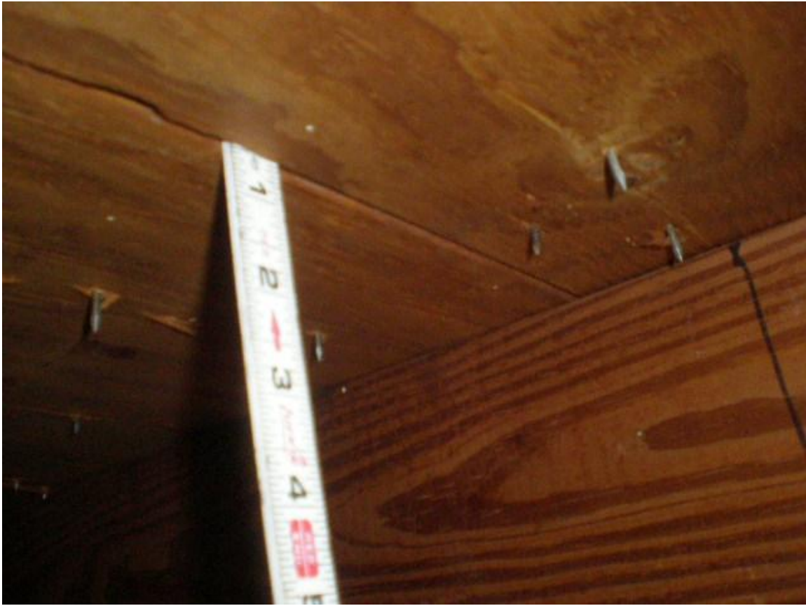
Roof deck staples
