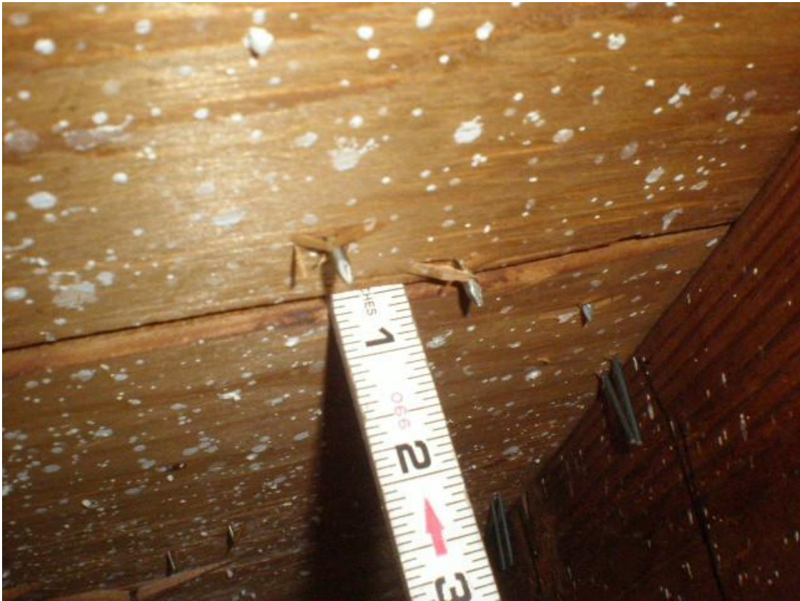
Roof deck staples
