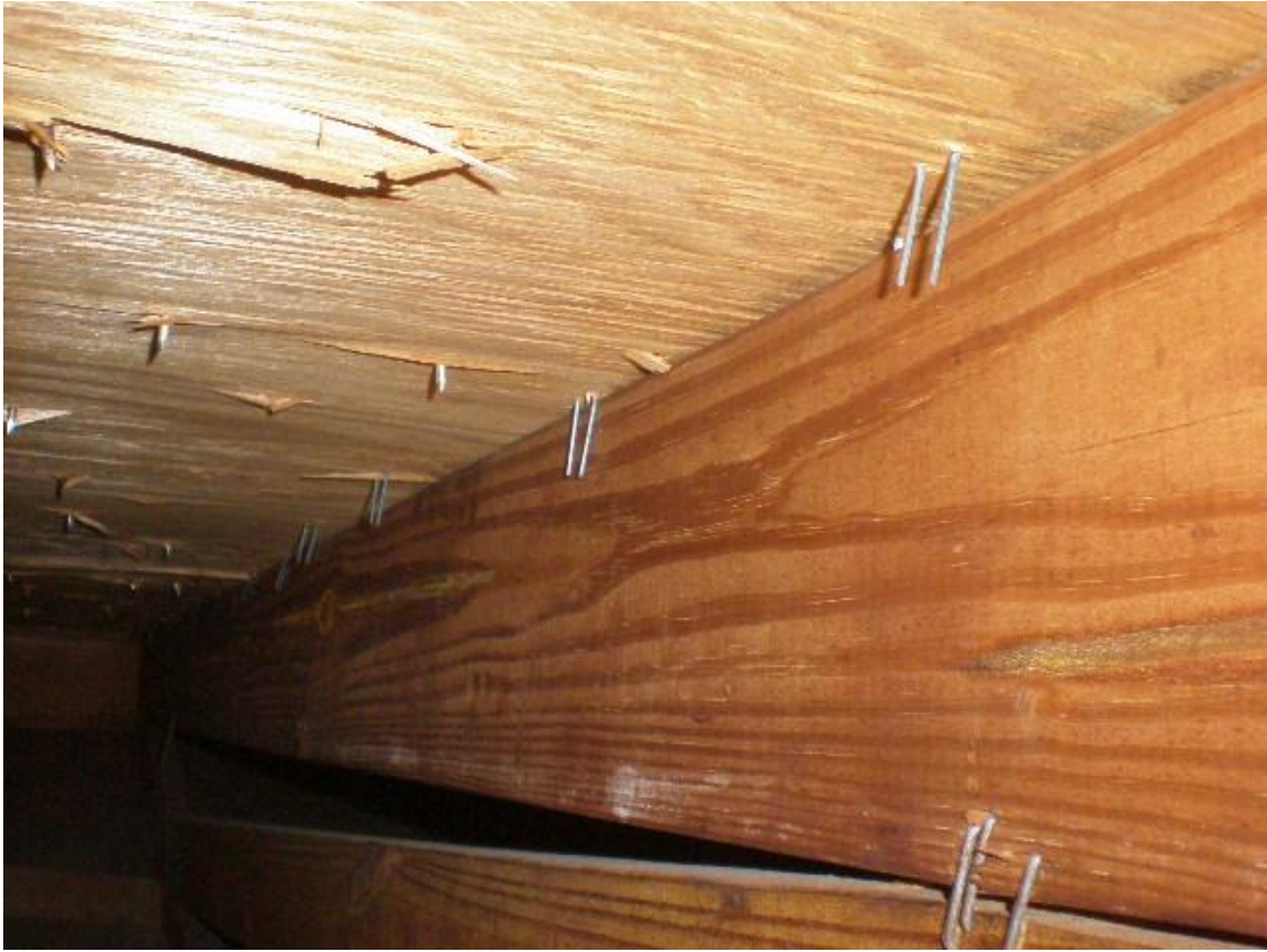
Roof deck staples
