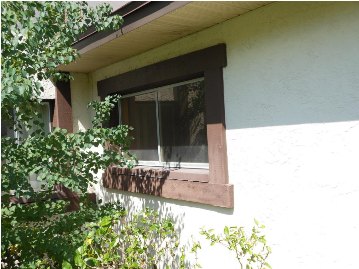
Unprotected openings
