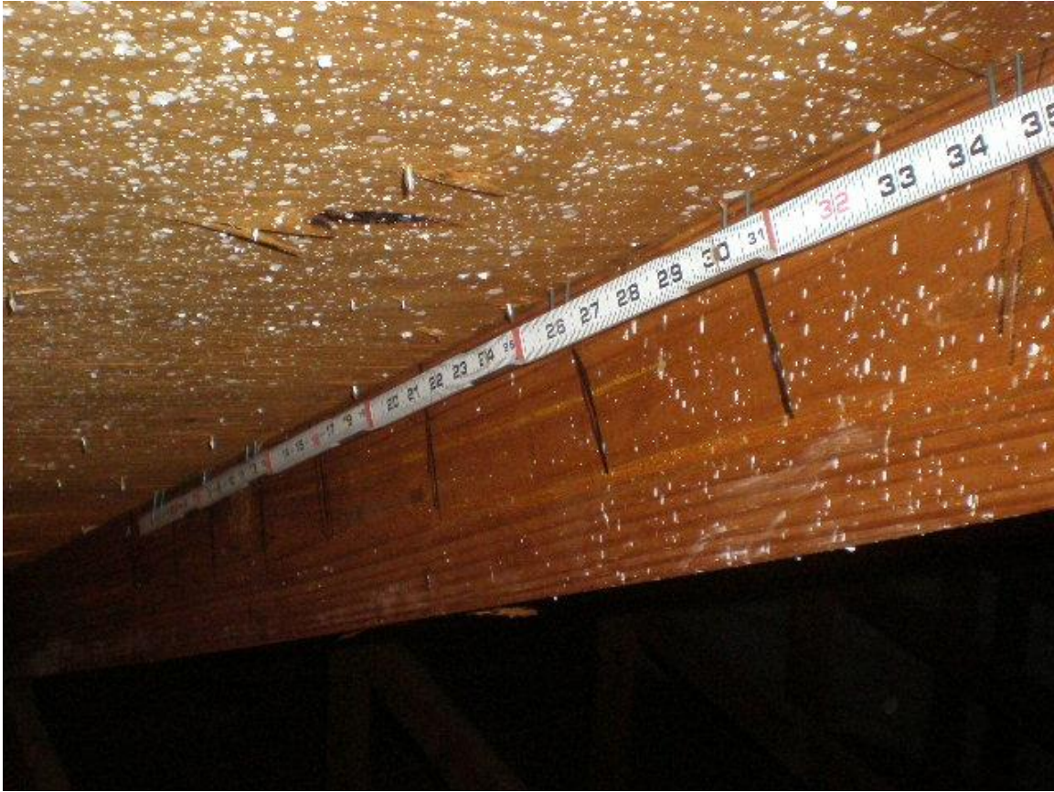
Roof deck staples
